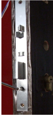
Install & fix the cylinder
